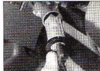
18.4b ... withdraw the lock cylinder
