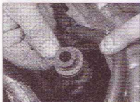
3.19 Inspect the mounting rubbers for signs of damage, and renew if necessary
