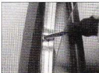
13.17a Slacken and remove the upper window guide retaining bolt ...
