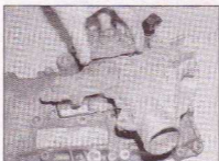
7.8 Withdraw the coolant pump from the timing cover – 1.0 and 1.2 litre DOHC engines (shown with timing cover removed)
