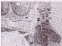
6.44 Apply a 2 mm diameter bead of silicone sealant to the joint between the cylinder block and cylinder head on each side
