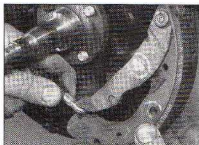
5.20 Engage the rear brake shoe with the handbrake cable, and locate the shoe on the backplate
