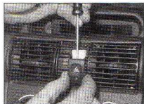
4.15 Removing the hazard warning light switch. Note the use of a piece of card to avoid marking the switch surround
