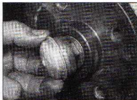
7.2 Remove the cap from the centre of the drum to gain access to the hub nut
