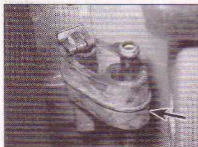
16.3 Check the condition of the exhaust system mountings (typical example arrowed)
